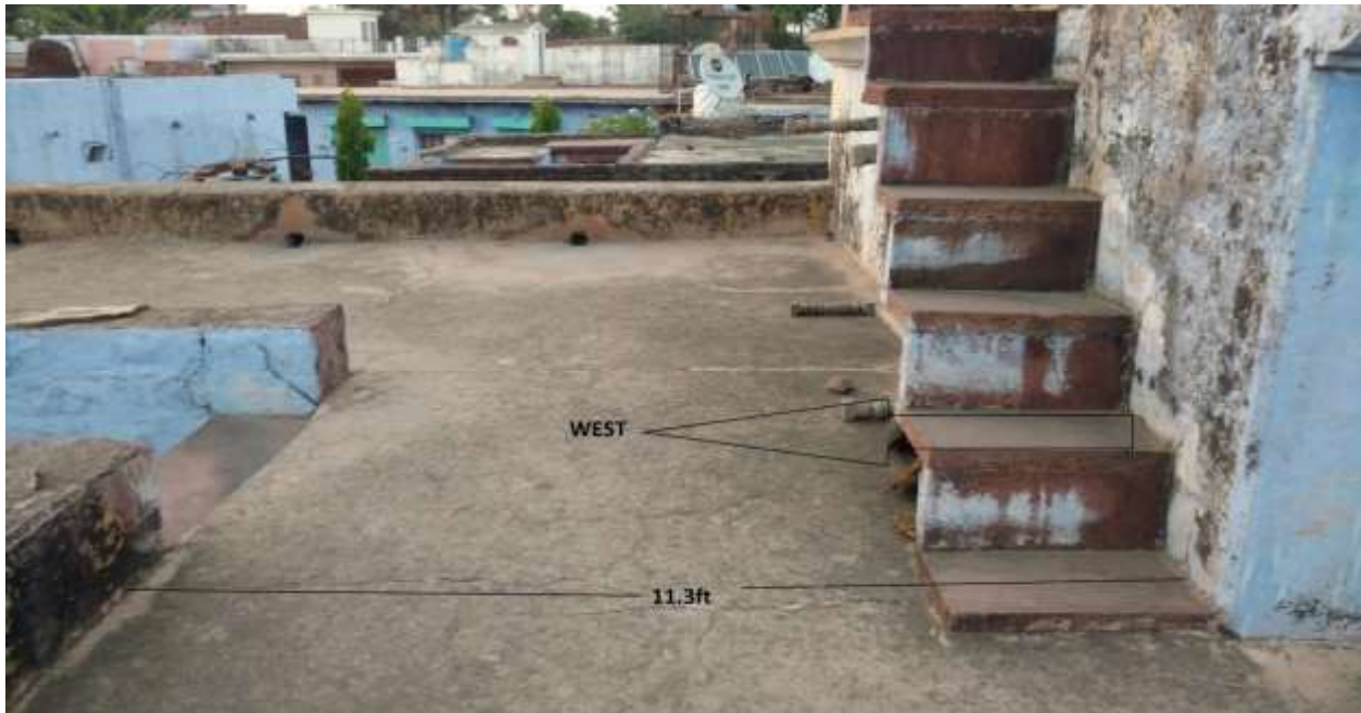
Figure 6 : West Side Protection Roof
