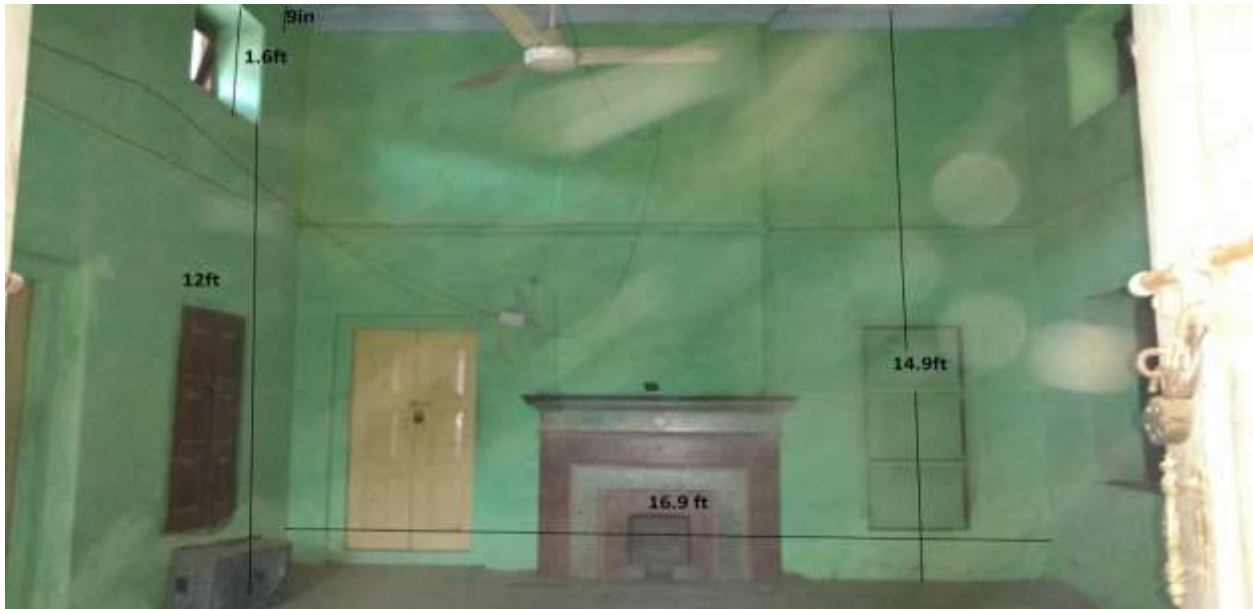
Figure 1: Passive building ( Area ,ventilation and chimney)
