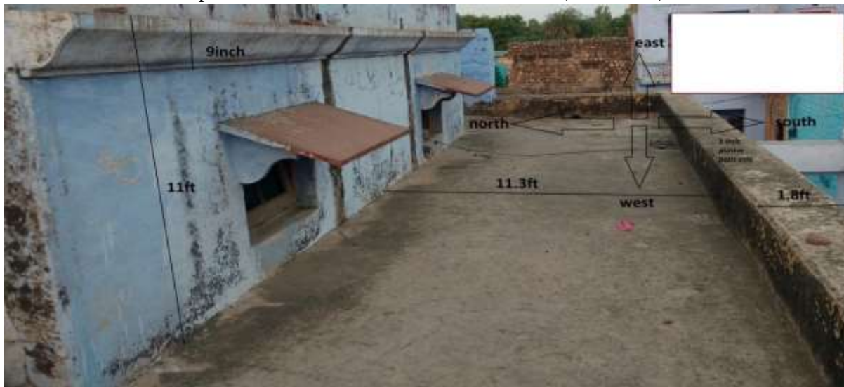
Figure 5 : South Wall protected by small room roof
