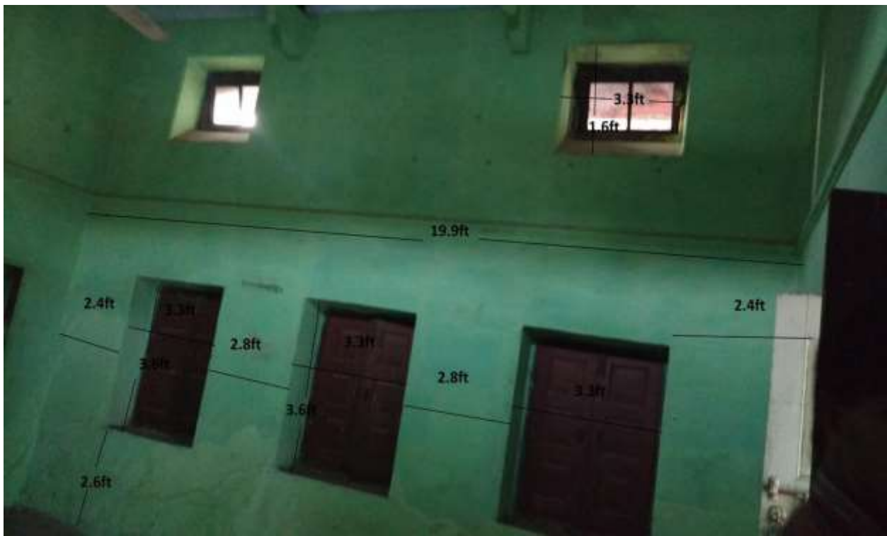
Figure 4 : North Wall (Window and Ventilation)
